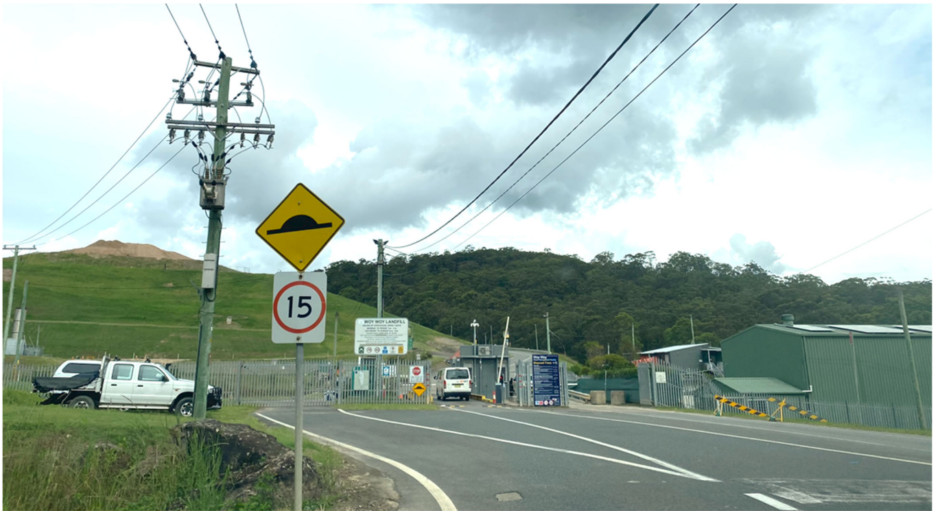
Figure 4.6 LCZ 3 – Infrastructure & Industry – Entry to the WMF Nagari Road
